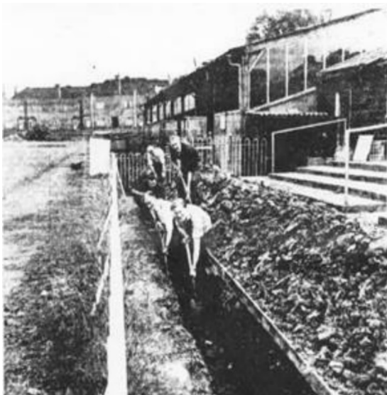
Supporters Club members digging the trenches for the installation of Floodlights.
